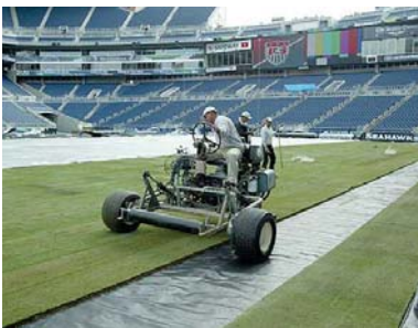
West Coast Turf installed a temporary natural grass field over the existing FieldTurf surface at Qwest Field, in preparation for the March 29, 2003, U.S.–Venezuela exhibition soccer match.
